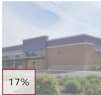
Building with Some Character and Landscaping; Parking in Front
